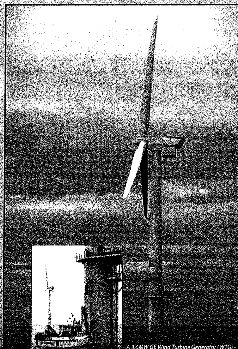
A 3.6MW GE Wind Turbine Generator (WTG) Arklow Banks, Ireland, courtesy of GE
