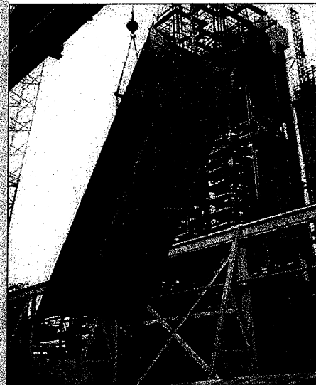
The vertical plates are lifted into place at a refinery in the western United States.
